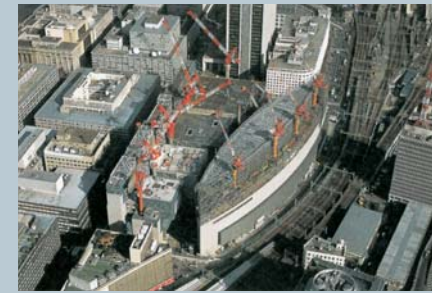
The Tokyo International Forum under construction; photo taken in Feb. 1995
